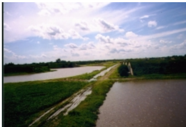
Water is directed to reshaped shallow basins by an open ditch with an individual check and turnout system
