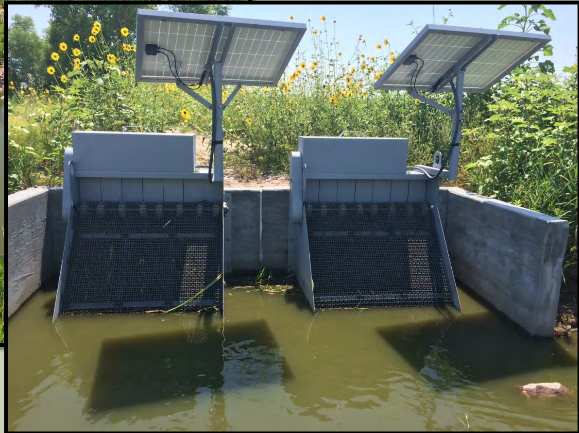
Installation of Carp Structures
