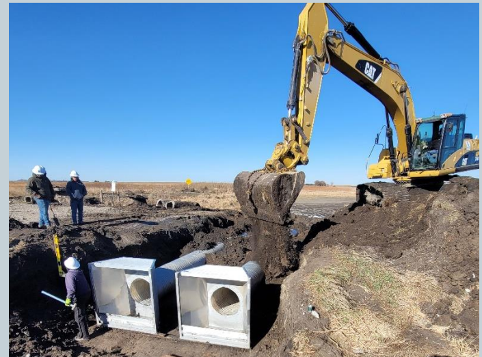
CNPPID helping with new culvert installment
